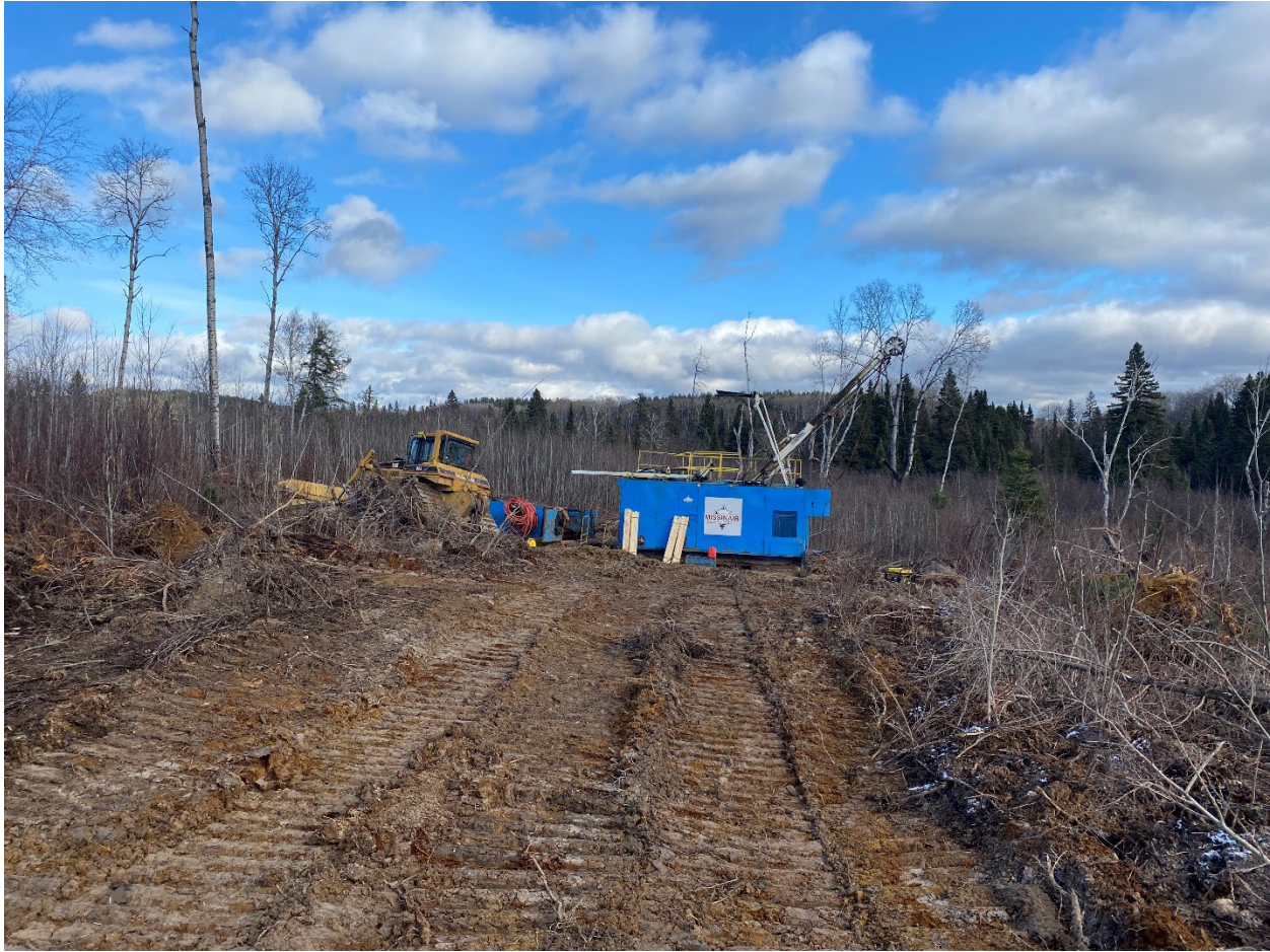
Figure 1 Drill set up on the first drill hole on Marriott Property.
