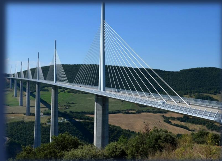
The Millau Viaduct in France was built using steel with 0.025% Niobium, which reduced the weight of the steel and concrete by 60%.
